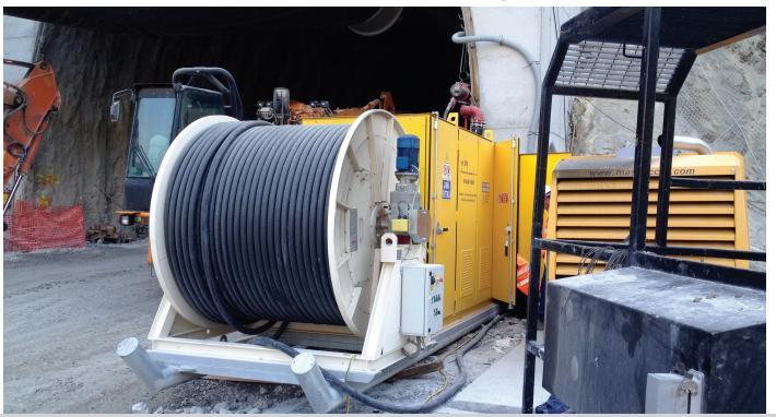
**TUNNEL TRANSFORMER SUBSTATION ON SKID** the tunnel transformer substation, operating on muddy grounds, is equipped with MV/LV cable reel and located on skid.
